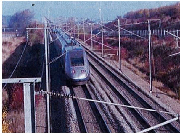
Figure 1.21: Catenary line, pantograph and rail return current to feed the train electrical traction chain. [13]
