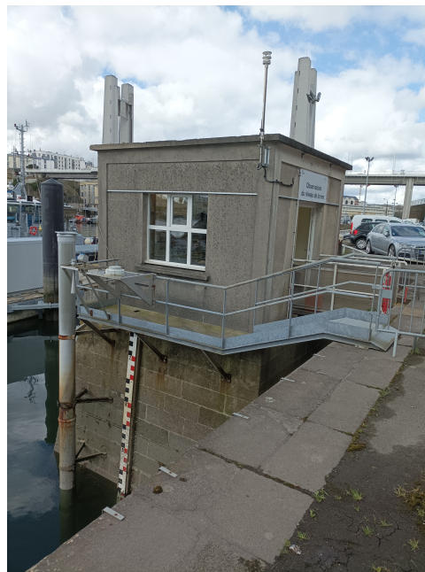
Figure 8.4: Photos taken during a visit of the SHOM, Brest, March 2024. Left: former Port-Tudy tide gauge. Right: current Brest tide house, with tide staff on the wall.
