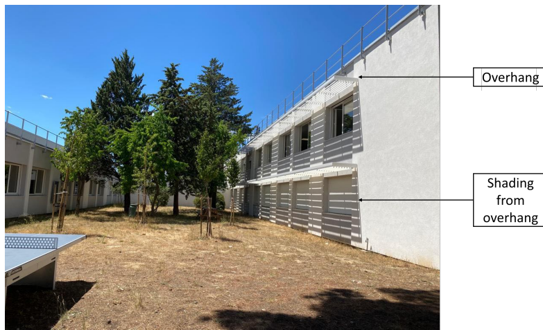
(C) Post-renovated façade on the south side
