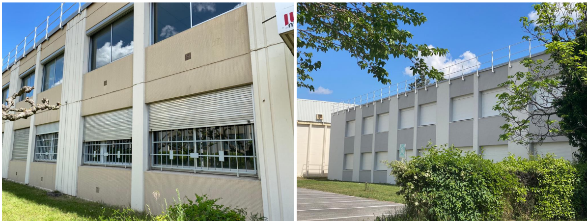
(A) Pre-renovated façade on the north side
