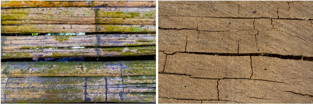
Figure I-6 - Wood in damp conditions (left) and with drying damage after swelling (right)
