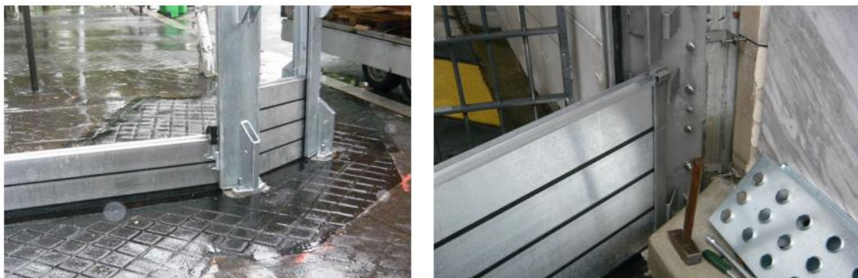
Figure III.E.8. Protections types batardeaux.
