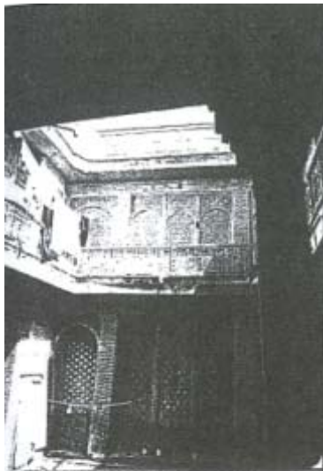
FIG(A8.2):View of the courtyard.
