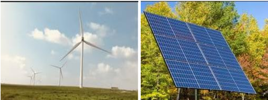
Figure 1.18: Pictures of installed wind turbine and solar panel samples
