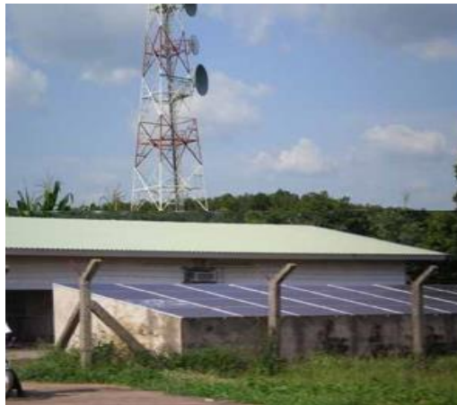
Figure 1.21: A solar PV powered base transceiver station [44]
