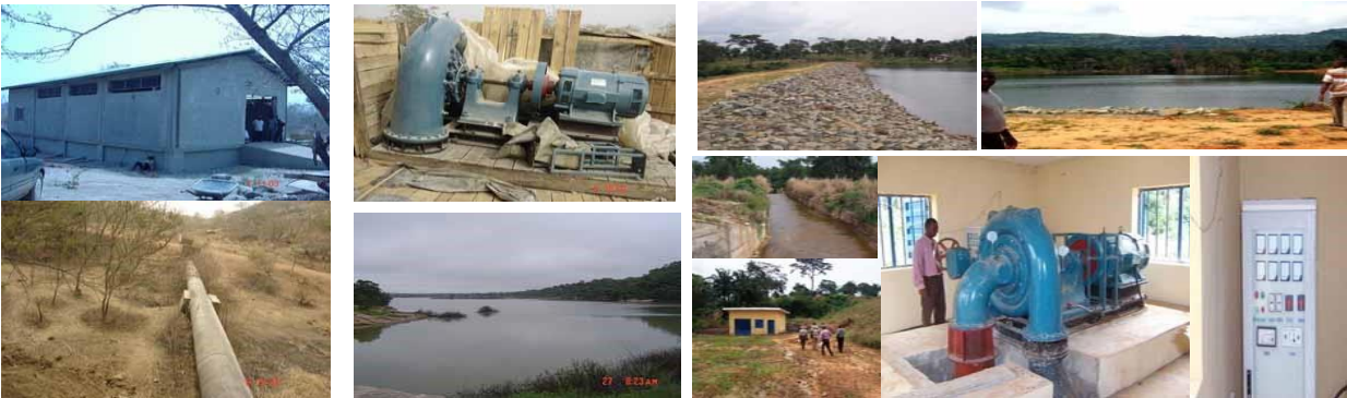
Figure 1.20: A 30MW small hydro development in Jos, Nigeria [44]
