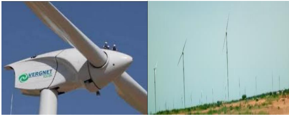
Figure 1.22: Pictures of Katsina wind farm project near completion in Nigeria
