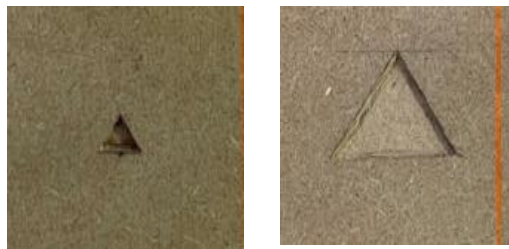
(b) Triangular cracks
