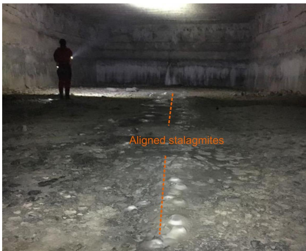
Figure 2. 7. Stalagmite growth near station CAU-2 aligns with fractures in the gallery’s ceiling. This growth pattern strongly suggests that fracture flow is a key characteristic for drips in Caumont Quarry.
