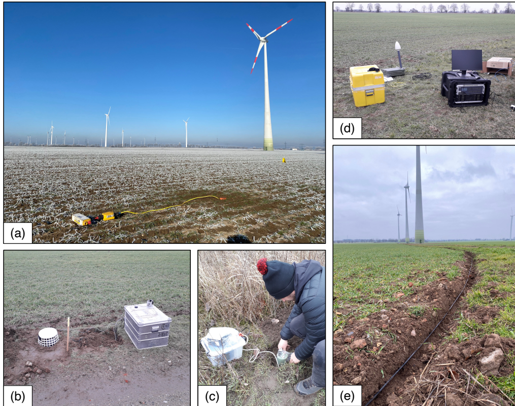
Figure 3.18: Deployment of various geophysical instrumentation in the wind farm. (a) A GS-One 3C geophone connected to a Reftek digitizer is seen installed in the foreground and an Enercon E-70 turbine standing 113m high in the background. (b) A rotational 6C station installed inside the wind farm, (c) 3C Broadband seismometer installation along the radial array, south of the wind farm, (d) An Alcatel Submarine Networks ‘OptoDAS’ interrogator at the start point of the cable, and (e) A 1km long DAS cable - Universal cable 8x50/125, OM2 fiber being deployed inside the wind turbine field.
