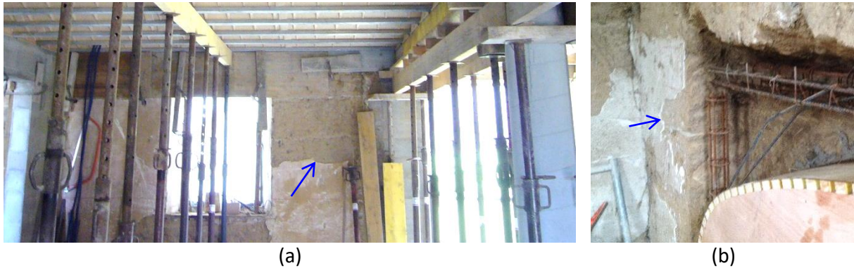
Fig. 2.8: Interior finishing plaster layer of traditional rammed earth buildings.
