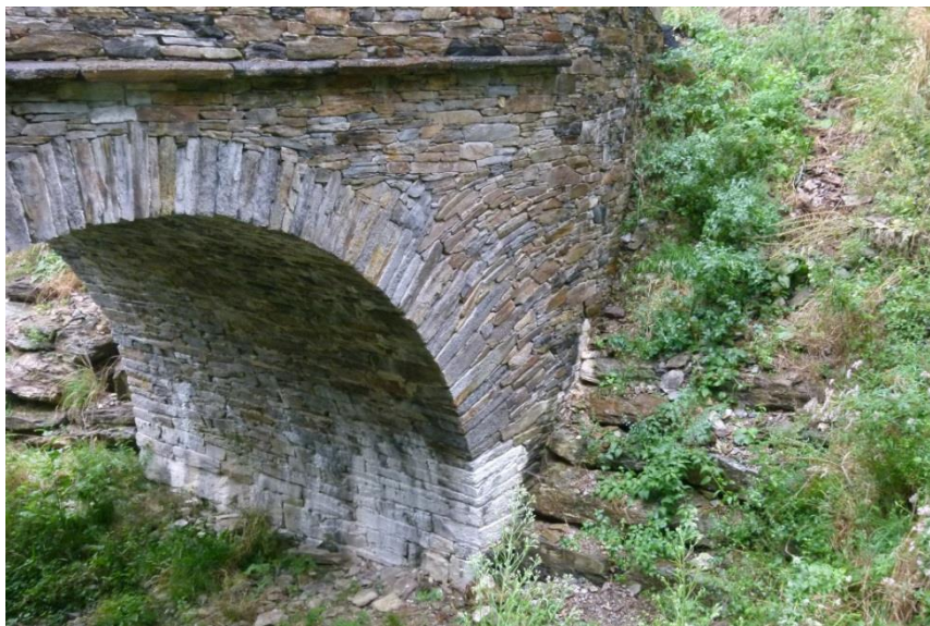
Figure 3: Focus on the haunches of Chaldecoste Bridge (Photo credit: P. Mc Combie)
