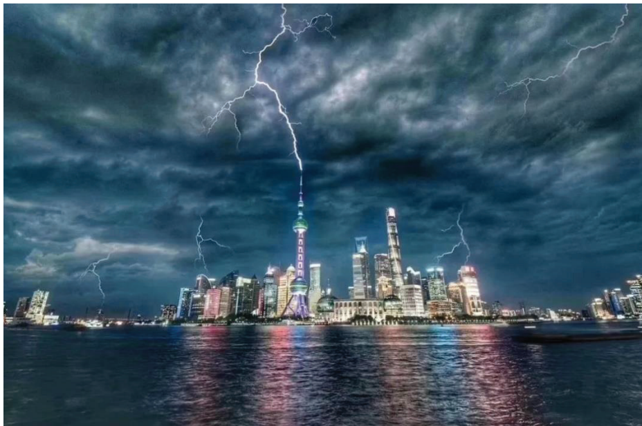
Figure 4.1.1. Photography of the Oriental Pearl Tower in Shanghai, China, struck by lightning.
