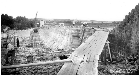
Figure 1: Repair of the post-failure Bouzey dam, 1895
