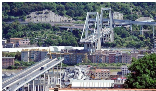
Figure 2: A photography of Morandi bridge post-collapse [23]
