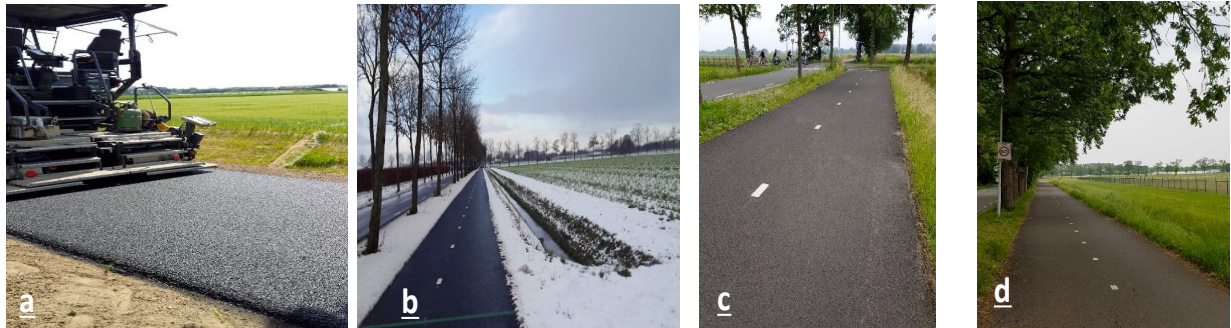
Figure 15: Example of cycling pavement built by mixing conventional bitumens with biobitumen issued from 3 different lignin biomass.
