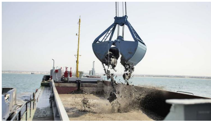
Fig. 29. Dredging sediment operation [179].
