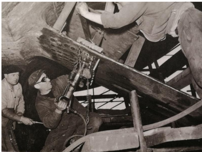
Rivetage du support Guepratte - © AHCNN/MHT
