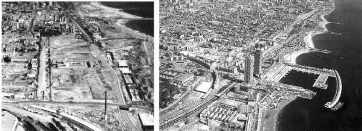
Barcelona: the coastal front under construction in 1990 and the Olympic village in late 1991
