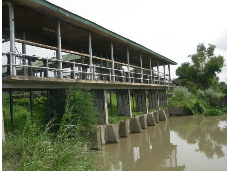
Figure 6-22 - Vanne de Sulipan (Macabebe).
