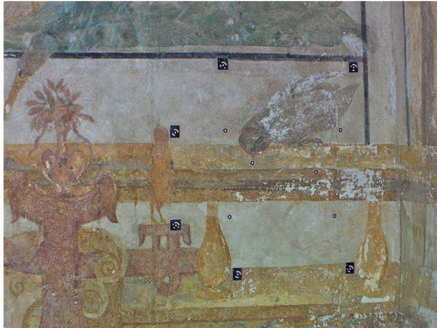
Figure 1.3: Flaking wall painting representing a bird on a balcony. Coded and uncoded targets are scattered around the area of interest.
