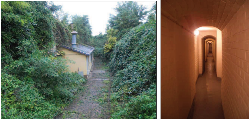
Fig. 3.5: Pictures of the outside and the inside corridor of the bunker J9, where the gravimetric observatory is located.
