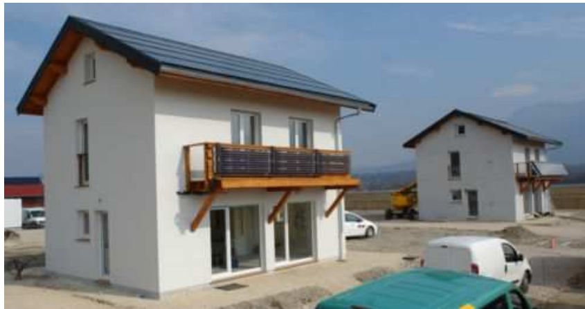
Figure 1.4 – Maisons INCAS (INES - Chambéry)
