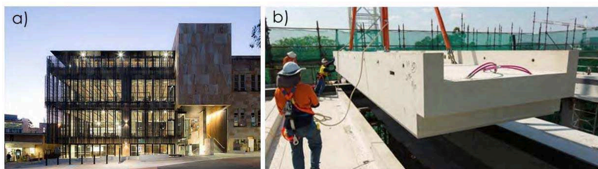
Figure 3. (a) Queensland University's GCI building (b) One of the 33 precast slag/fly-ash-based geopolymer concrete floor parts ( www.geopolymer.org )
