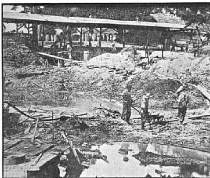
View from Coffey Dam, Looking Across the Rosin Mine or Pit, Where Ten Feet of Water has been Pumped Out
