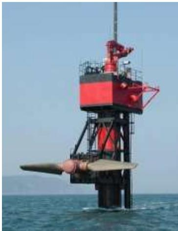
Figure B-2. SEAFLOW émergé
