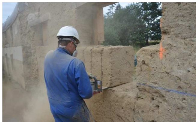
Figure 37. Portions of cob wall cut thanks to a rock chainsaw
