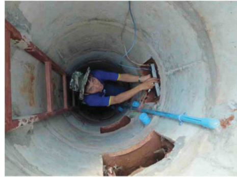
FIGURE 5 | Root scanning in access shaft (5 m deep) in Lao PDR (Maeght, 2012).
