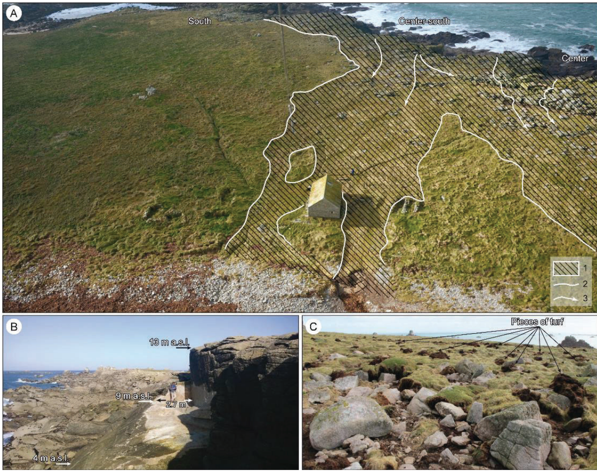
Figure 2-11. Field evidences of large submersion and block quarrying on Banneg Island during winter 2013–2014. (A) is a kite oblique aerial photograph taken on February 18, 2014, during survey 3 (credits: J-P. Boivin) where 1 is the flooded area, 2 is the limit of the flooded area (discontinuous debris line and limit between bended / stood grass) and 3 illustrates the flow direction. Photograph (B) illustrates the largest quarrying socket inventoried after the winter 2013–2014. Photograph (C) is a ground oblique view of the block field mixed with large pieces of turf.
