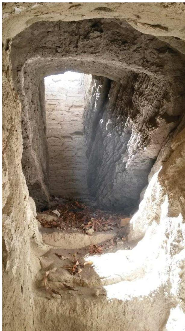
Figure 22 : Typical shaft well (Lumbrera) in Pica area
