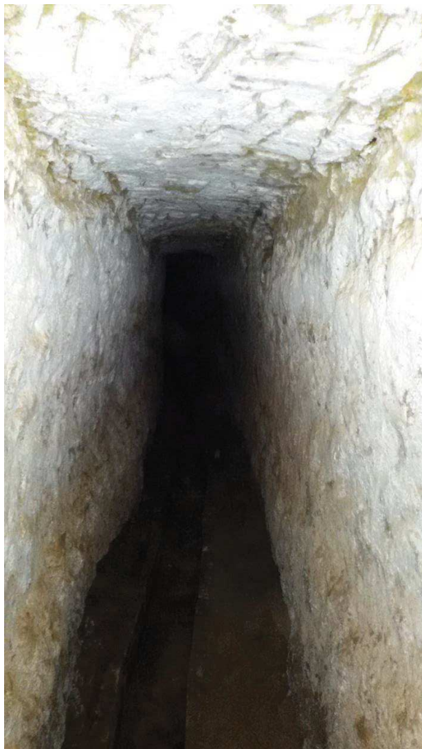
Figure 19 : Baked clay tiles channel in Comiña socavon.
