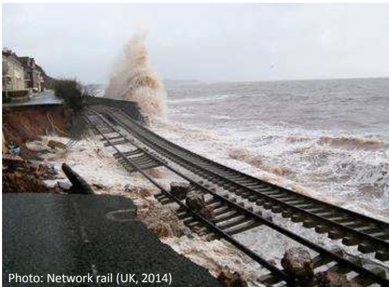
Photo: Network rail (UK, 2014)
