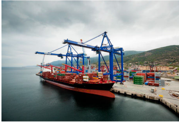
Figure 1.3: Loading and unloading crane
