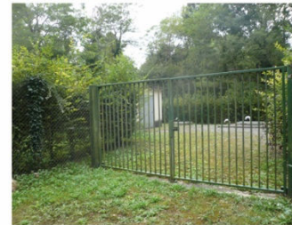
Cesson (77) - Station d'épuration
