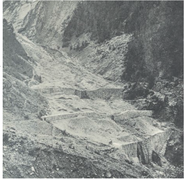
Figure 1.3 – Headwater-moraine-retention-dams in the Ravin des Arandellys (74 – FRA.) (Eaux et Forêts, 1911a)
