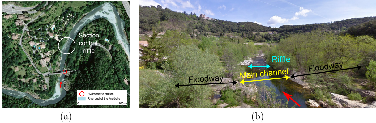
Figure 2.10 – Views of the hydraulic controls of the Ardèche River at Meyras: (a) from above, Géoportail database; (b) downstream of the bridge from the left bank, Google Earth view.
