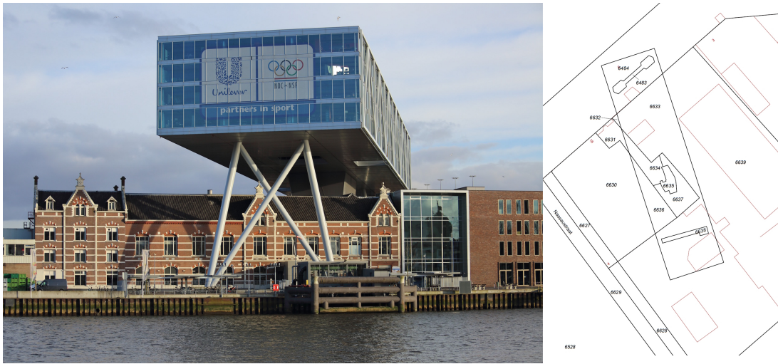
Figure 1.1: Example of a problematic situation where 3D cadastre would be of help and 2D maps fail. The two building footprints overlap and are too complex to be represented in 2D. Image taken from (Biljecki et al., 2015b).
