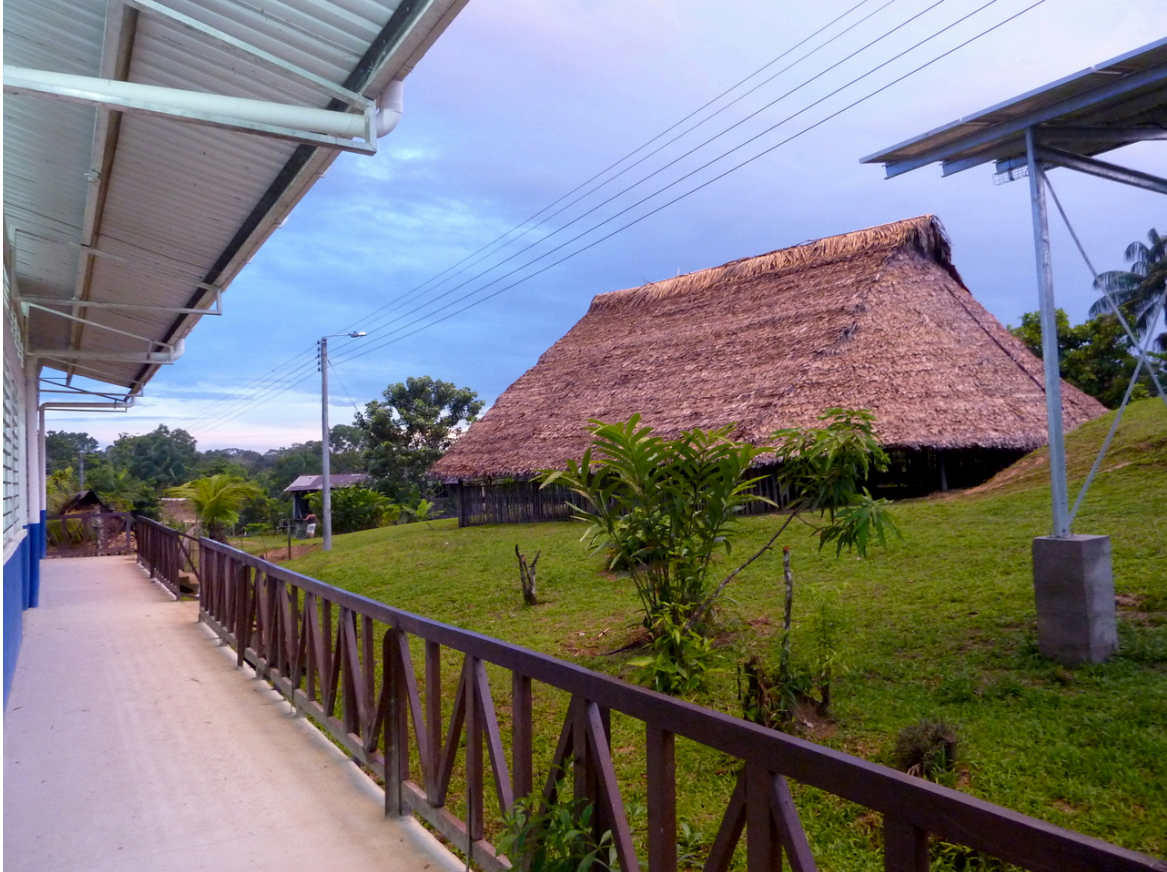
FIGURE 6. View from the lower school building on the communal maloca at the heart of San Martín de Amacayacu
