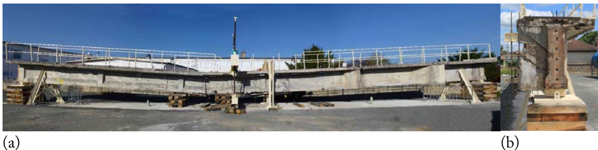
Figure 2-46 : (a) Bending test of the Clerval beam -2014; (b) profile of the Clerval beam, with prestressed cables.
