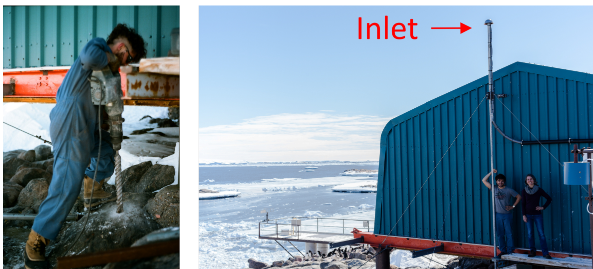
FIGURE 5.17 – Left: Quentin Perret making the mast hole. Right: Amaelle Landais and I standing next to the mast where the inlet is fixed. The blue building is the "labo glacio".
