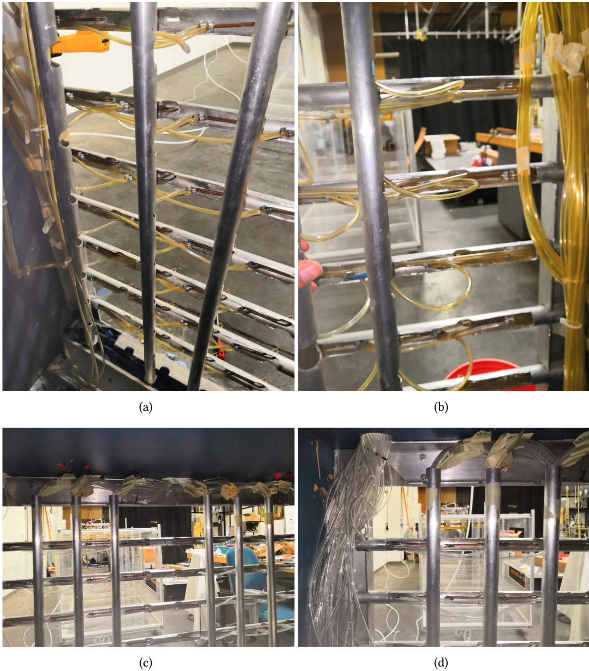
Figure 10.2 – a-b) Illustration of the cuts required to access the injectors notice that the old piping was yellow, whereas the new piping is transparent.
