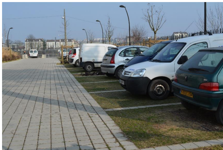
Figure II.16: Parking perméable de Villeneuve-le-Roi
