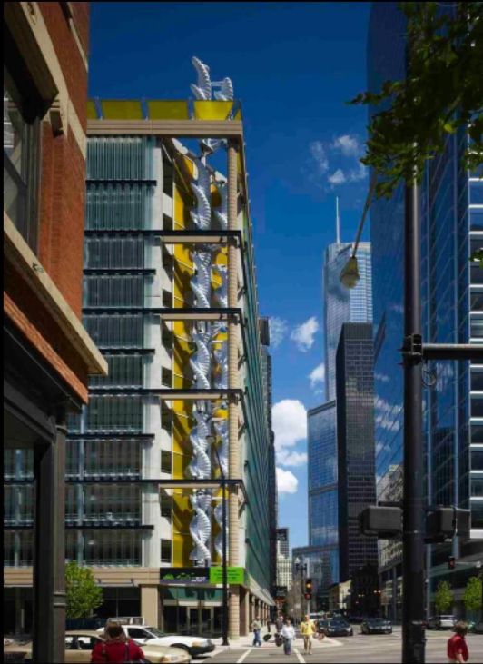
EXISTING BUILDING INTEGRATED WIND HARVESTING DEVICES - VERTICAL AXIS WIND TURBINE
