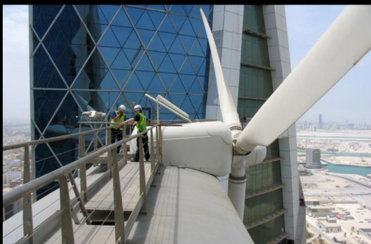
EXISTING BUILDING INTEGRATED WIND HARVESTING DEVICES - HORIZONTAL AXIS WIND TURBINE
