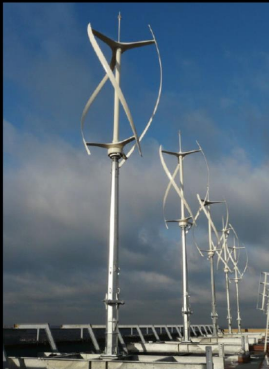
EXISTING WIND HARVESTING DEVICES - VERTICAL AXIS WIND TURBINE
