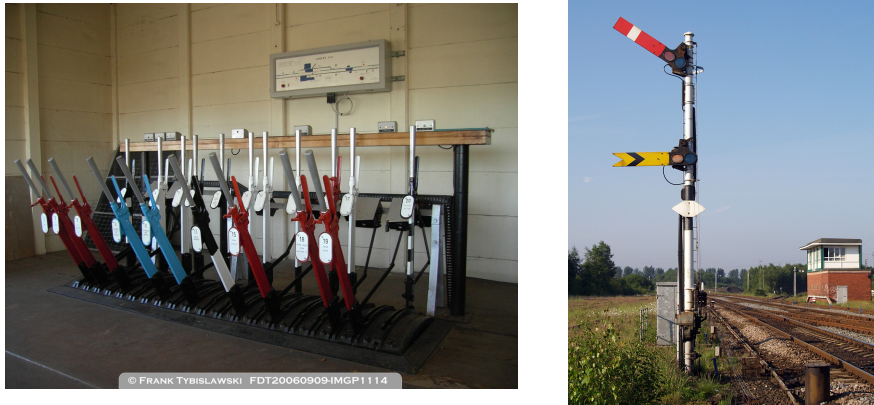
Figure 2.3: a) Signalling tools, b) Track-side signals
