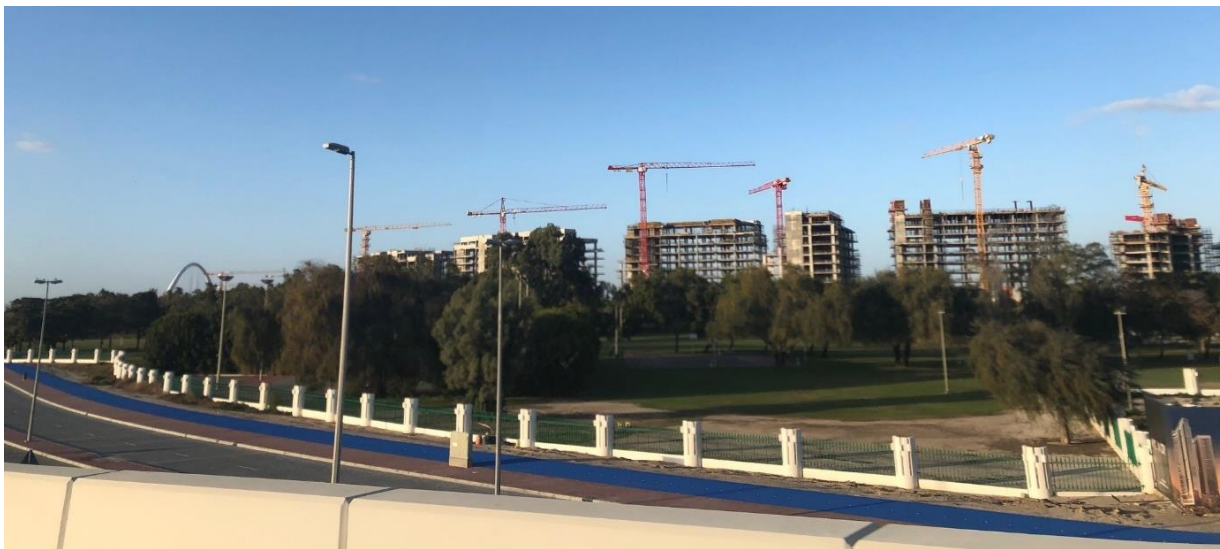
Figure 69: Al Safa Park from Sheikh Zayed Road.
