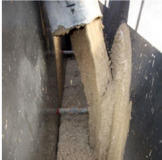
Figure 1-9 Self-compacted earth (source: Mathieu Neuville)
