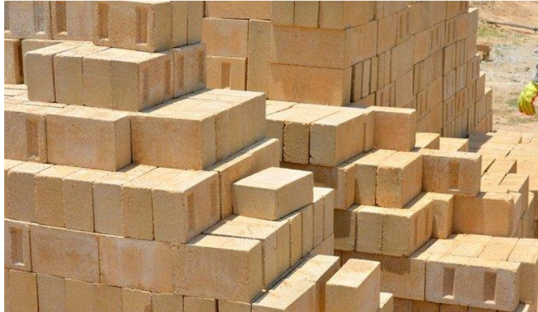
Figure 1-8 Compressed earth blocks produced for the construction of model houses in Karaveddy, Manmunai West, Batticaloa. (Source: Jaime Royo Olid, EU Delegation 2017)
