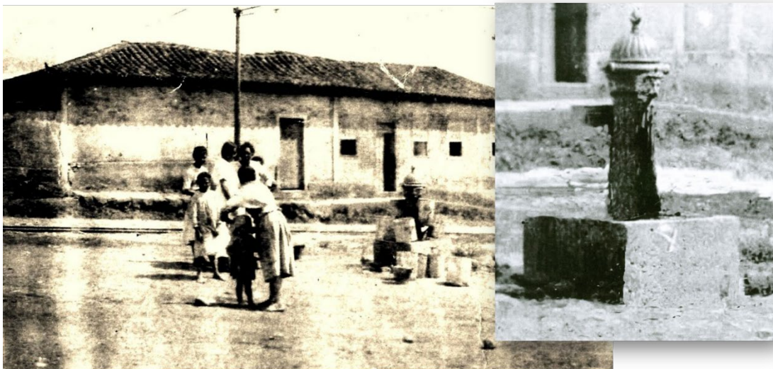
Figure 5 - Public fountain installed in 1885 at Praça Dr. Jorge.
