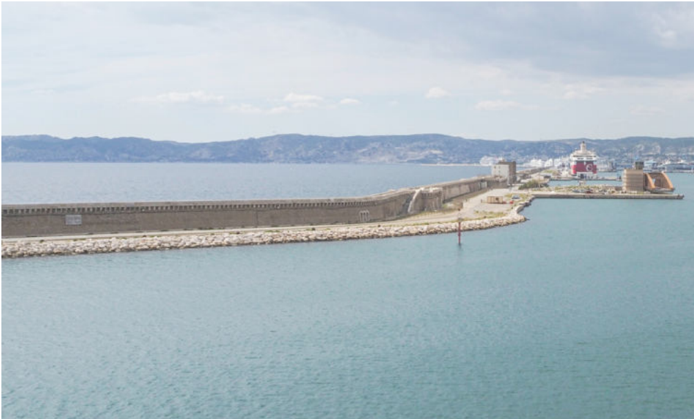
Fig. 133 - The Digue du Large in Marseille is a large walkway on the water, within to the port system, used for logistic operations but included in a process of progressive pedestrianization. It also represents an extensive barrier from sea waves (picture by the author, 2021).
