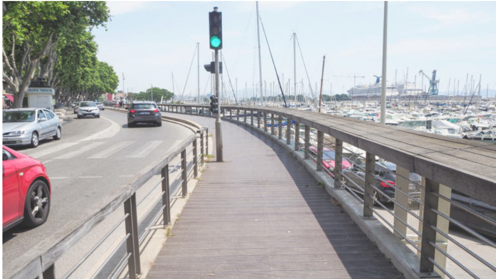
Fig. 146 - Above, the small pedestrian promenade in L'Estaque, in the 16th Arrondissement of Marseille, runs alongside the numerous local nautical clubs. Below, Pointe Rouge beach, nearby the Calanques area: the area has undergone interventions for functional implementation (pictures by the author, 2021).
