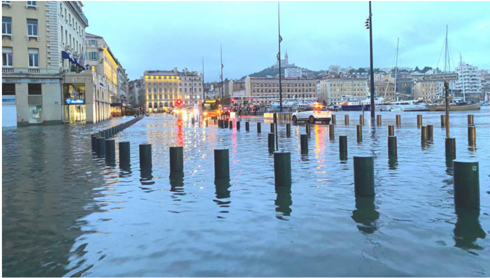
Fig. 4 - The devastating flash flood of May 2021 totally submerged the Vieux Port of Marseille (source: M. Geay / Gomet' Média, 2021).
