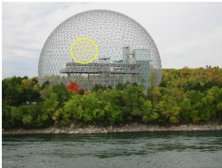
Fig 4.23 The United States' pavilion in Montreal, designed by Buckminster Fuller inspired the structure of C_{60} . The yellow circle (AD) is centred on one of the pentagons necessary to bend the structure. Source: Cédric Thévenet, CC BY-SA 3.0, Public Domain.
