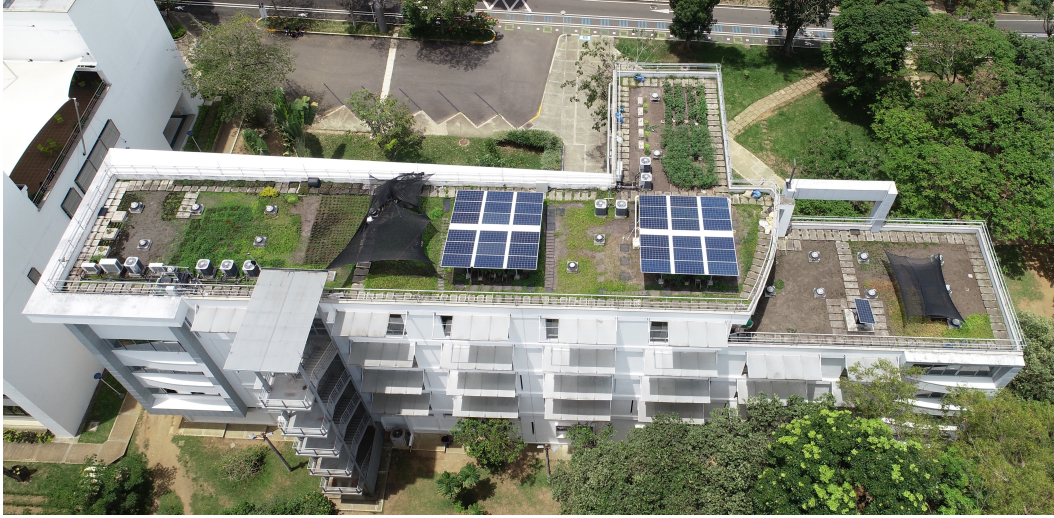
Figure 3.3: Top view of the PV system on the EEB-UIS rooftop.
