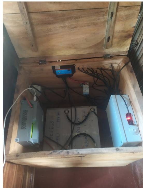
Figure IV.7: Interconnection module mounting and installation on the field.
